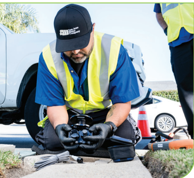
Installation of advanced metering infrastructure (AMI) at San Jose Water that enables smart meters to provide near-real-time usage information.
