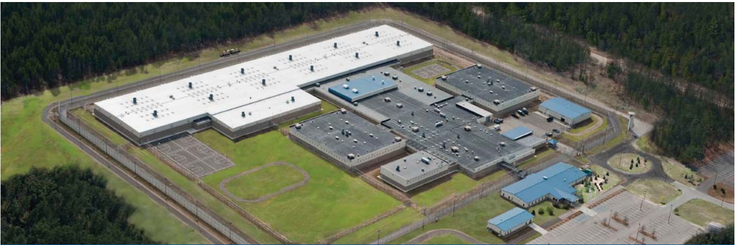
NORTH LAKE PROCESSING CENTER (MI) 1,800 BEDS
