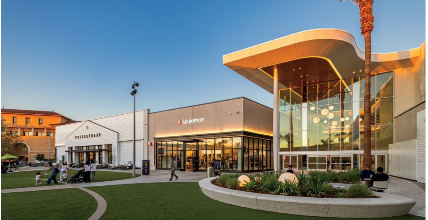
▲ Brea Mall , Brea, CA
