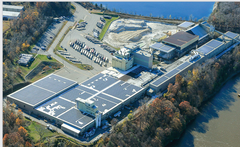
Saint Gobain's CertainTeed Gypsum facility in Buchanan, NY is pictured. Photo Credits: Saint-Gobain North America
