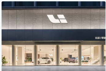
Store renovation and refurbishment projects
